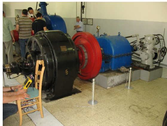
Fig. 8. Balancing and alignment adjustment of the generator assembly
