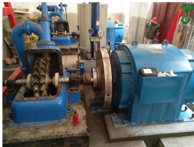
Fig. 9 Alignment adjustment of the new generator and turbine
