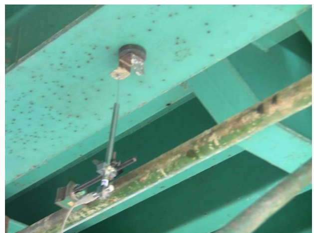
Fig. 5 Displacement transducer LVDT (W50) set on the transverse girder
