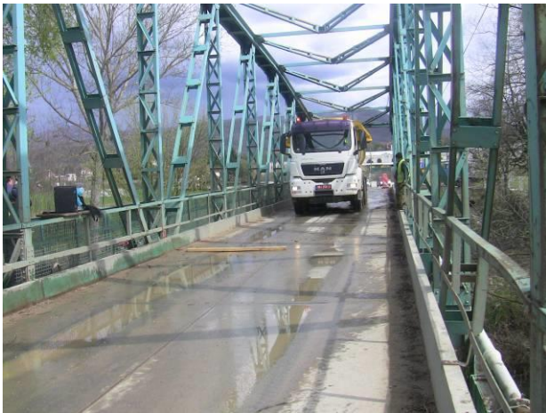
Fig. 6 Passing of vehicle during measuring of dynamic parameters of the bridge
