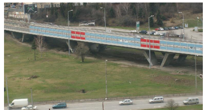
Fig. 7 Acoustical measure – noise barrier, real set-up
