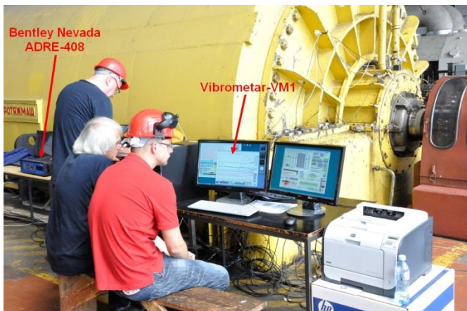
Fig. 9 Vibrometar-VM1 measuring vibrations at turbine-generator set A2-TENT-A (210MW) 05-07-2013.
